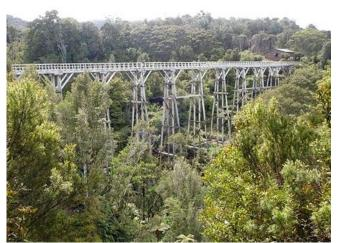
The Percy Burn trestle viaduct was the longest and highest of four such viaducts along the logging tramway. *Image DOC* Total length 125 metres (410 ft) Height 36 metres (118 ft) Opened 1923 Closed 1928
