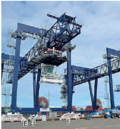
The new RMGs
