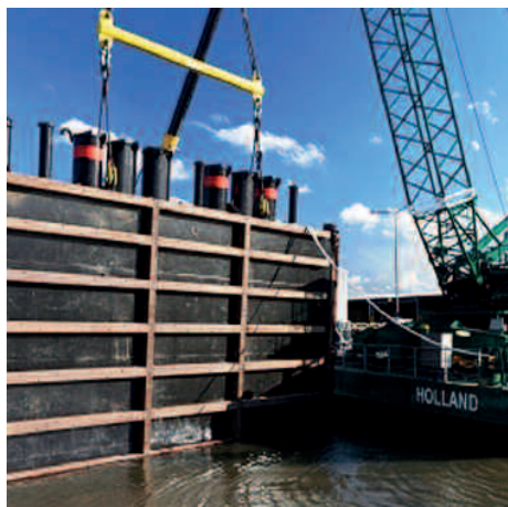
The new inner lock gates are installed at King George Dock
